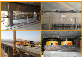
Only the extreme low height CLP-cylinder fits in this confined area to lift the construction. The V-82 needle valve is used to control cylinder speed during lifting and lowering.
