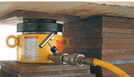
Only the extreme low height CLP-cylinder fits in this confined area to lift the construction. The V-82 needle valve is used to control cylinder speed during lifting and lowering.
